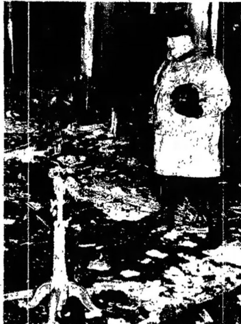
VIEWS RUINED BOWLING ALLEYS —Mike Mickok, bowling coach and manager of the alleys, holds a warped, blistered ball in the rubble of Archbold gym's ground floor, where the fire is believed to have originated.
