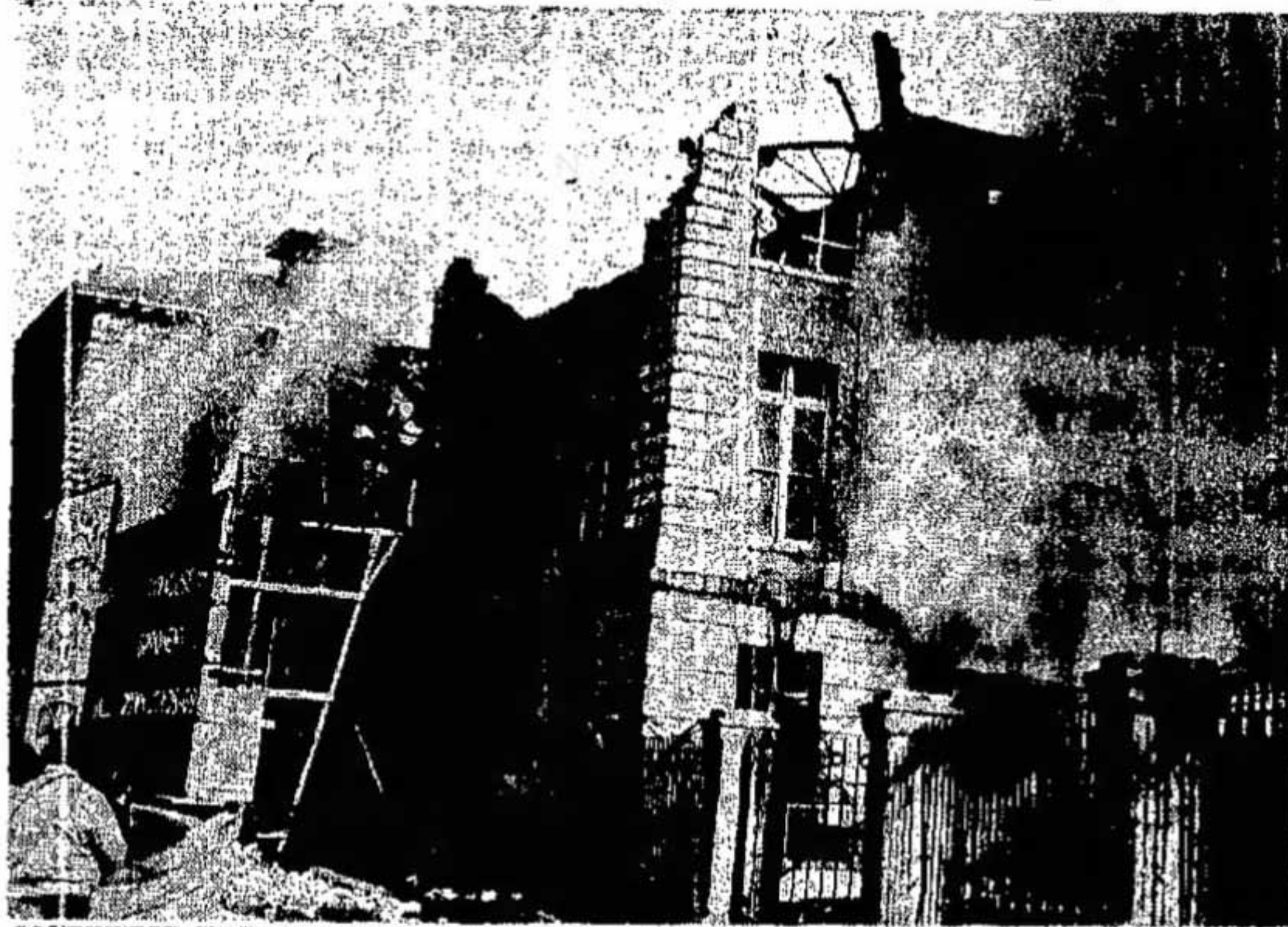
SOUTHWEST SIDE —Part of the gymnasium facing the stadium is shown in this picture. Locker rooms are on second floor, with visiting team rooms in the basement corner.
