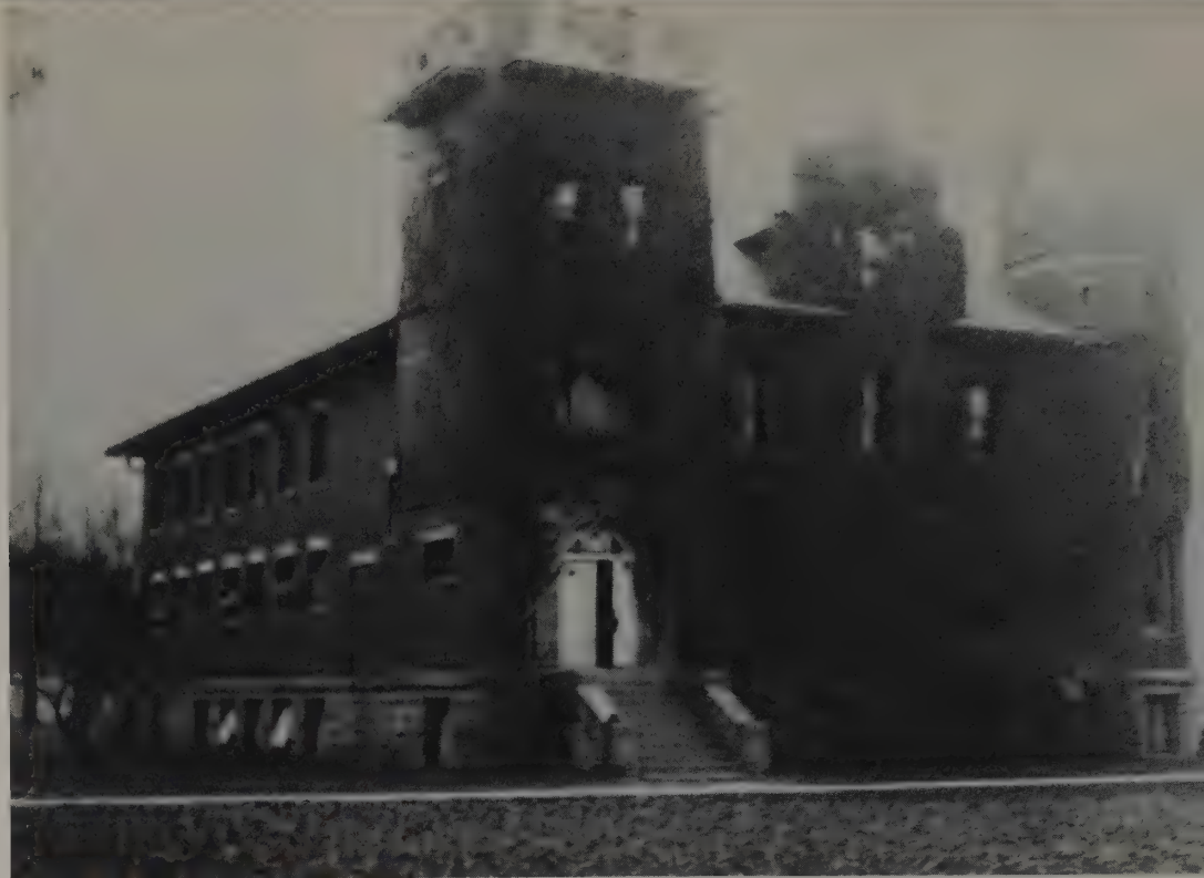
Present-day Olde Union Theatre prior to renovation.
